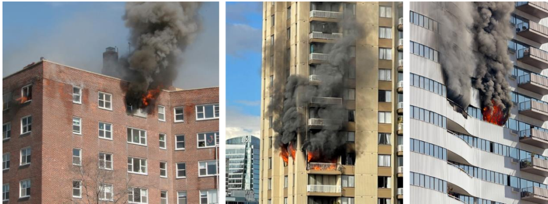
Fig. 1. Smoke and fire behaviors outside the building from different views [41–43].
