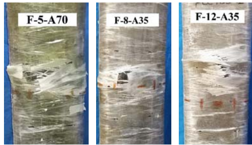
(b) Rupture of the FRP tubes of FCCSCs
