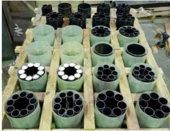
Fig. 3 Formwork for casting concrete
