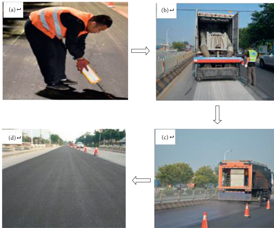
FIGURE 4: Construction of sand fog seal: (a) pretreatment of the old pavement; (b) surface grinding; (c) sand fog seal spraying; (d) preservation after sealing.
