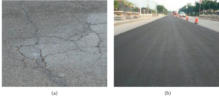
FIGURE 6: Pavement surface: (a) before WEB sand fog seal treatment; (b) after WEB sand fog seal treatment.
