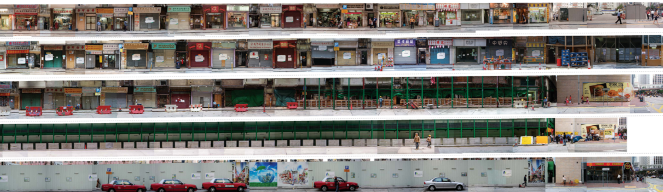
4 | A visual documentation of the 5 stages of the demolition of Lee Tung Street photo by Tse Pak-chai
