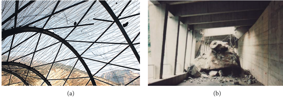
FIGURE 2: Failed rock shed. (a) Flexible rock shed. (b) RC rock shed [1].
