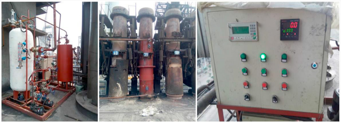
Fig. 2. Photographic image of experimental apparatus: (1) Circulation system; (2) APHE at outlet of coke oven gas; (3) Control and data collection system
