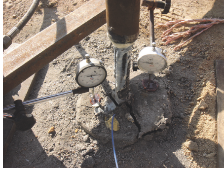
FIGURE 9: Cracks on anchorage body at failure.
