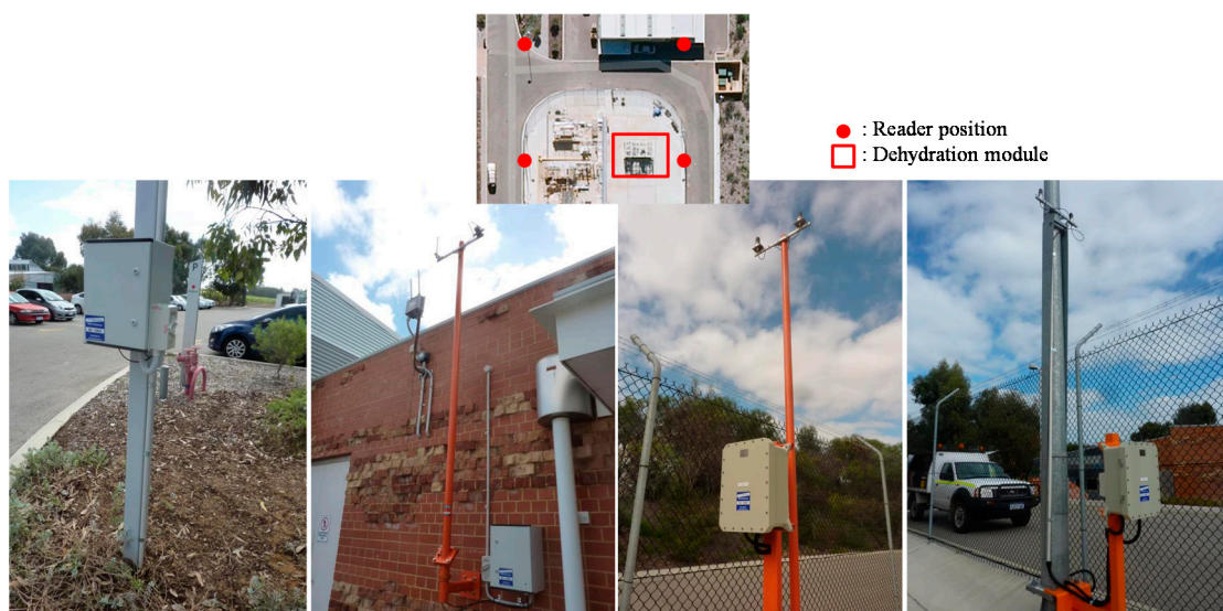
Figure 9. Four fixed RFID readers around the dehydration module.
