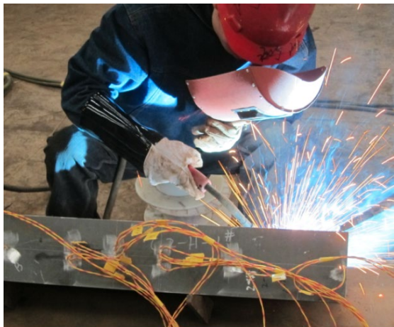
a) Gas metal arc welding (GMAW)
