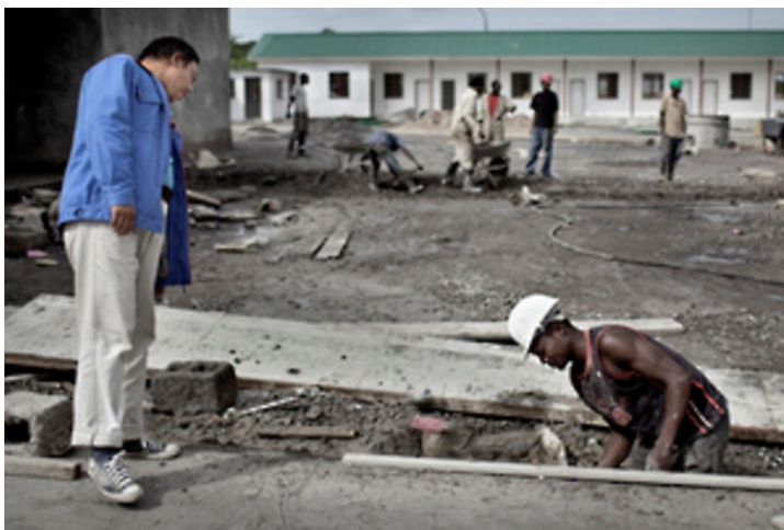
A Zambian does construction work at China Luanshya Mine as a Chinese manager looks on. China Luanshya Mine is one of four copper mining companies in Zambia operated by the Chinese parastatal China Non-Ferrous Metal Mining Company. From the HRW report.
