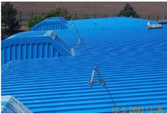
Figure 2.7 Typical cable system (Glasgow Caledonian University, 2005)
