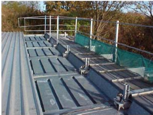
Figure 2.1 Purlin trolley systems (Glasgow Caledonian University, 2005)
