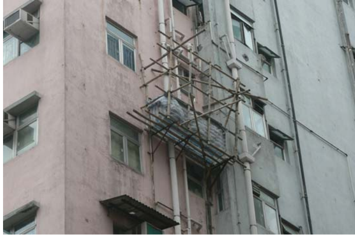
Figure 4.1 Photo of a bamboo truss-out scaffold supported by steel brackets on a typical residential flat
