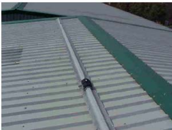
Figure 2.8 Typical track safety system (Glasgow Caledonian University, 2005)
