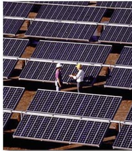
A 210-kW flat-plate PV array that is used for grid support.
