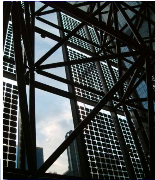
Figure 9: The interior view of the Skylight BIPV system of the Wan Chai Tower in Hong Kong
