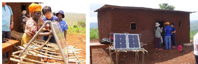
Fig. 1. The original (2015) Household-Based Solar System. Panels are attached to a frame of PVC pipes to create a foldable, movable structure (Left). The panels are brought out for charging when necessary (Right)
