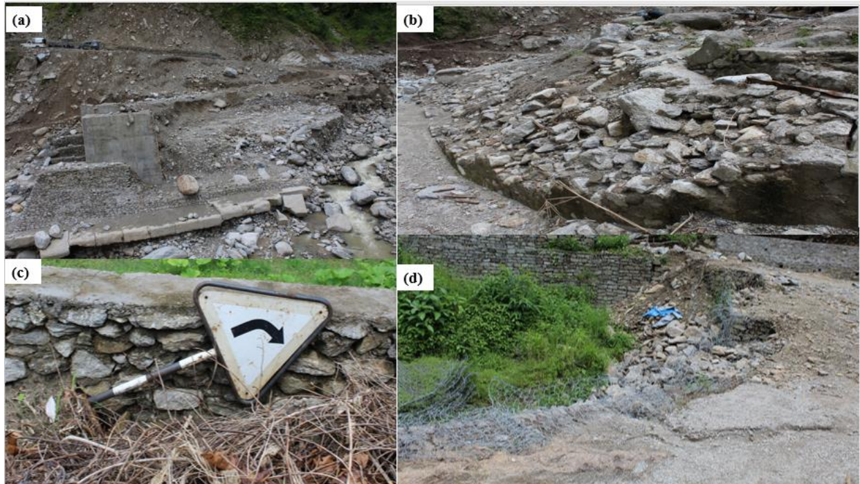
Fig. 5 a) Road damage due to flash flood; ~2 km long stretch was washed away with no indication of road alignment; b) exposed subgrade of the road; c) damaged sign post along the road; and d) damage to the gabion wall
