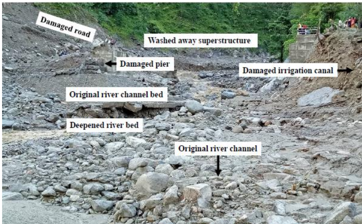
Fig. 3 Debris flood from the stream due to flash flood in the bridge site
